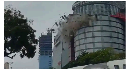
Explosion in Taichung City department store leaves 4 dead, 26 injured
